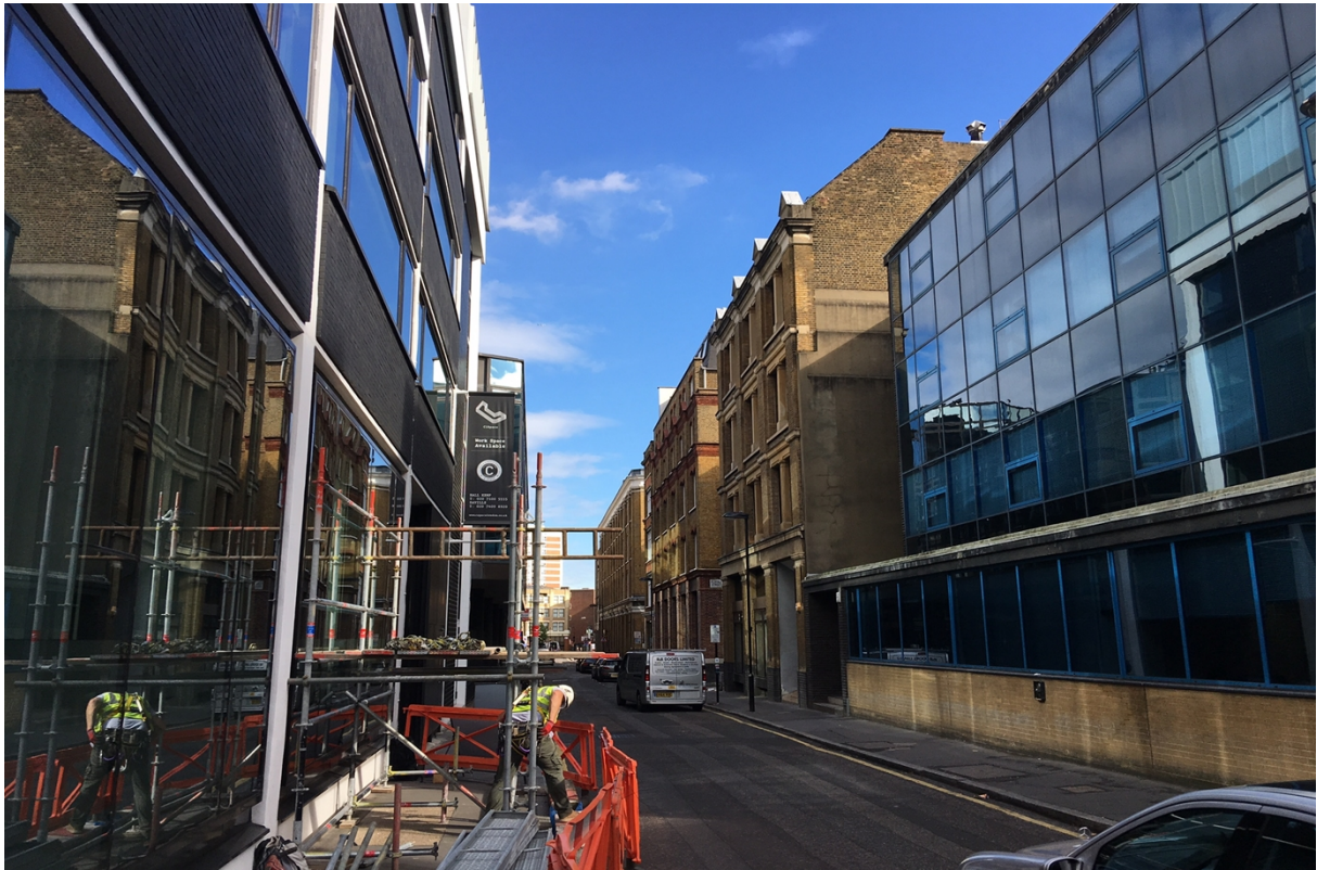
Fig 5: Looking North along Tabernacle Street
