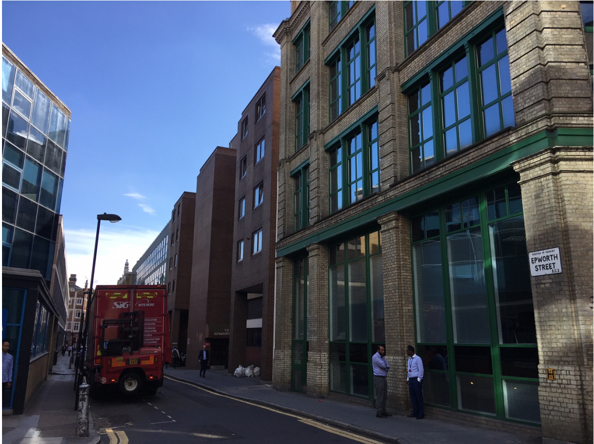
Fig 6: Epworth Street looking east towards residential flats at 10 Epworth Street
