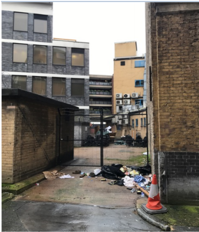
Figure 7. View of the service yard from Platina Street (sub-station to left)
