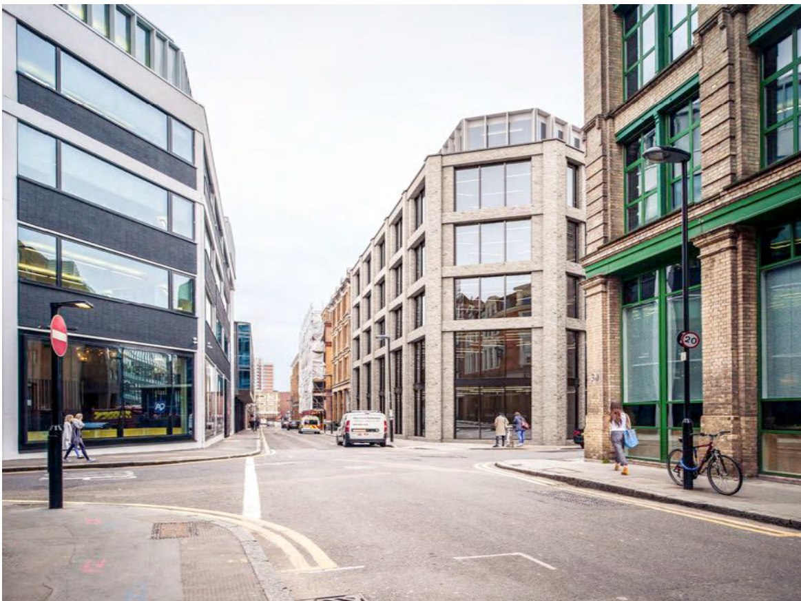
Figure 13: Looking north along Tabernacle Street
